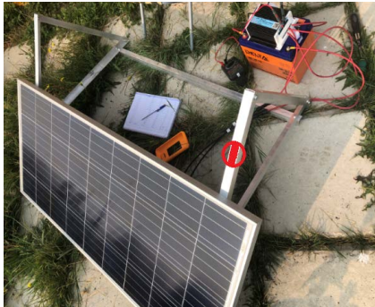
Fig. 3. The solar power plant 150 W.
