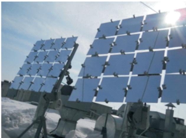
Fig. 1. Mirrors of heliolighting system
